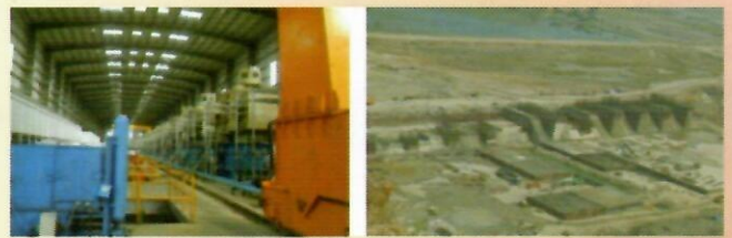
Pattiseema Lift Irrigation Motors Spill Way Construction of Polavaram Dam
